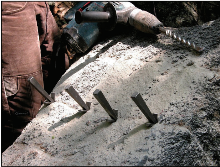
A rock rifted, drilled and ready to be split.
