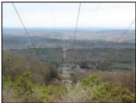
PSE&G wants to widen this corridor and double the height of the towers.
